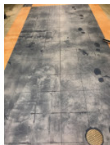
Stripped of finish
