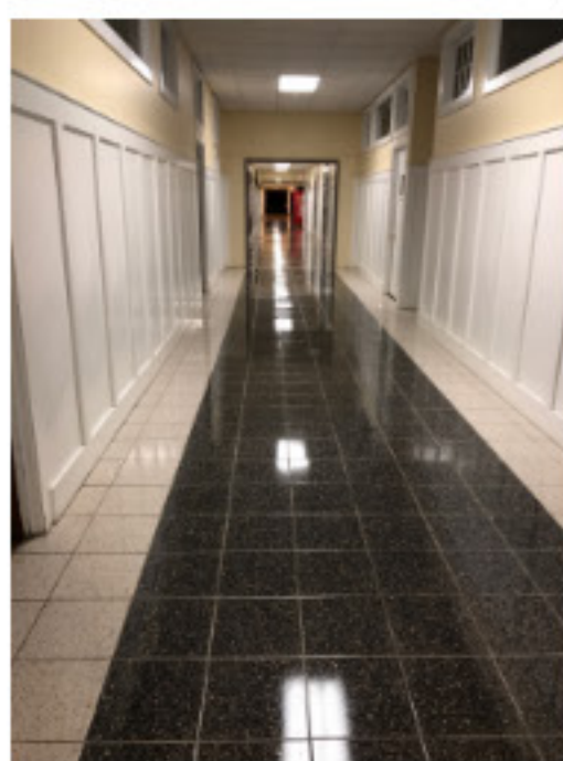
Ceramic tile floor after refinishing
