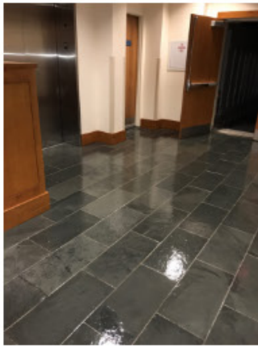
Bluestone floor after refinishing
