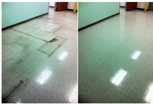
VCT Tile floor before and after refinishing.
