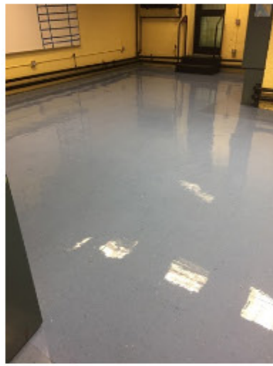
VCT floor - after wax has been reapplied
